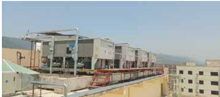
Supervision Air Cool Chiller 400 Ton Installation in Islamabad.
