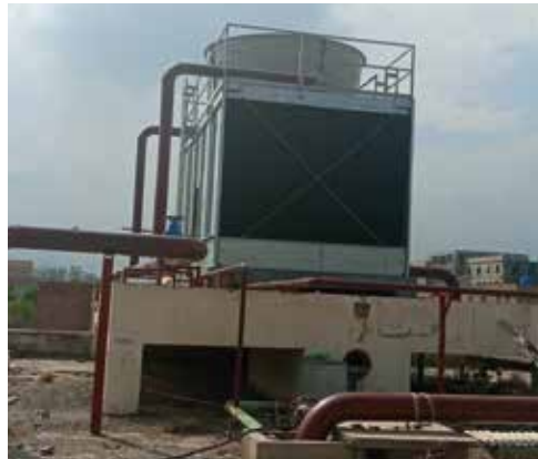
Supervision Cooling Tower Project Completed.
